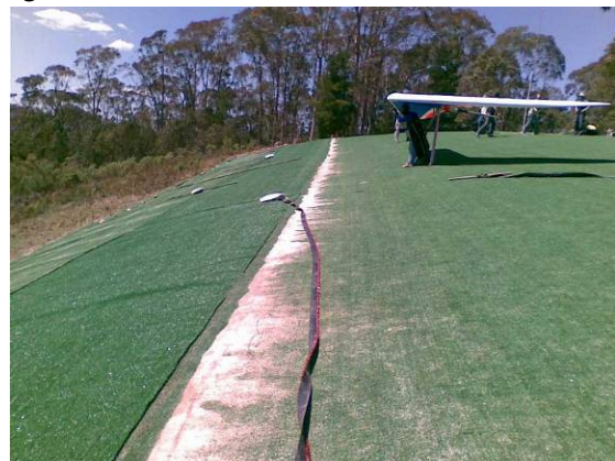
New surface with extension under construction
