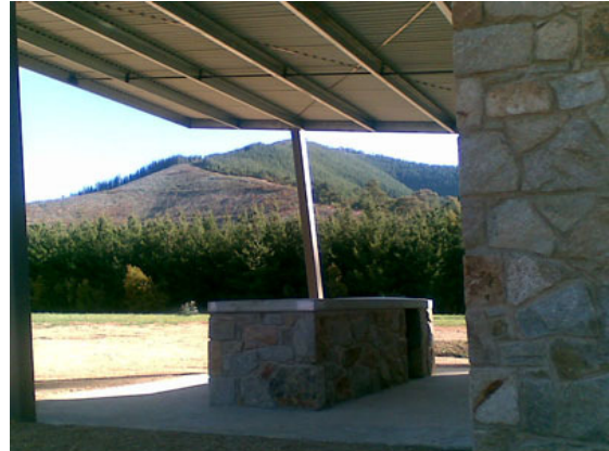
BBQ, shelter and toilet block with a view of Mystic.
